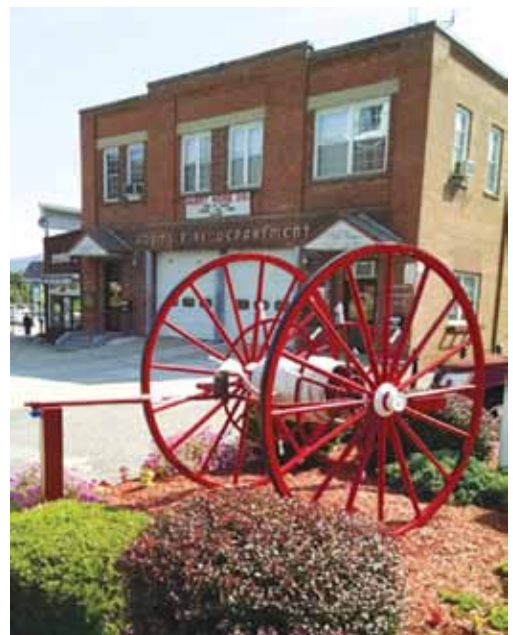
Right: Restored 19th-century hose cart on display next to the Fire Station
