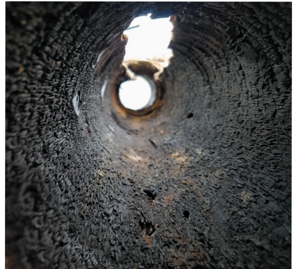
The charcoal remains on the pipe's burnt interior lengthens its lifespan and aids in water purity.
